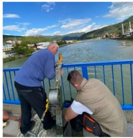
Figure A3 -2 : Placing the winch on the bridge
