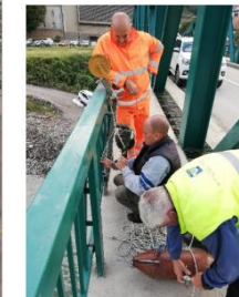
Figure A3 -3 : Connecting torpedoes
